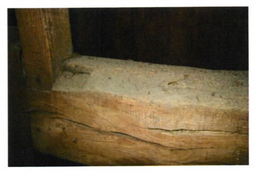
The tie beams have been used to support hangers for the First floor. These will be referred to again later.
