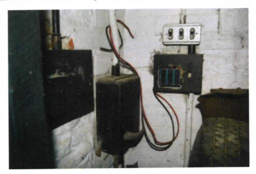
The whole of the electrical installation is substandard and it will be necessary for you to rewire the building to your own requirements.
