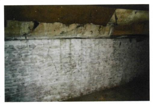
There are no signs of recent movement, and as these cracks have developed during the last two hundred years or so, they are not considered to be the result of recent movement and therefore do not require any immediate action. However, it would be prudent to restore the ground level on the South side to its original height. In particular, this would reduce the amount that is washed away by passing traffic.
