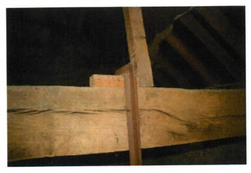
At the East end, there is a beam against the East wall. This is supported by posts rather than being fixed to the walls. The posts show an active infestation of wood-borers.
