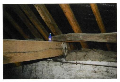
The roof has an ancient timber frame with major tie beams at eaves level. On these are posts supporting tie beams and purlins. The timbers show signs of infestation by wood-borers, but no recent activity was observed.
