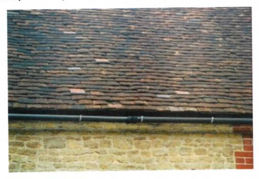
The tiles sag at the eaves. This is presumably due to the tilting battens having rotted. Some repairs are necessary.
