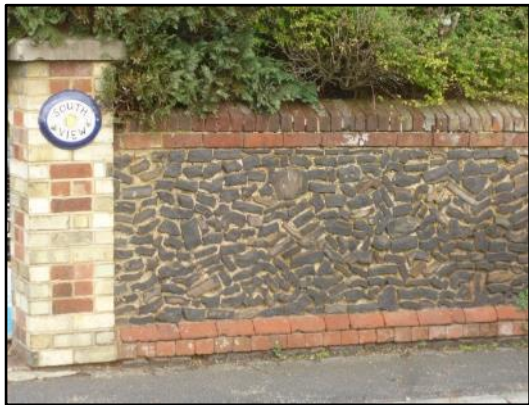
Brickwork with local Ironstone
