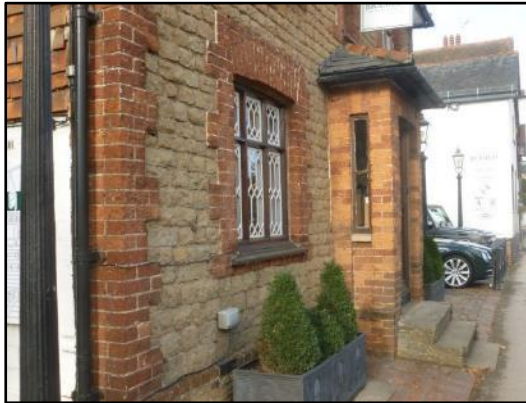
Bargate stone with brickwork
