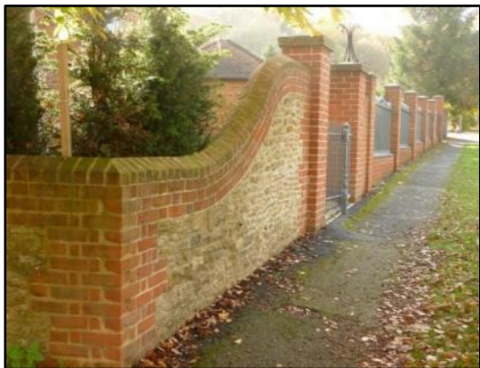
Brickwork with Bargate Stone
